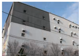
Ariake No. 3 ABC Center (Ariake, Koto-ku, Tokyo)
