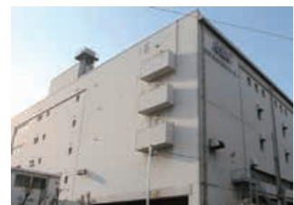
Ariake No. 1 ABC Center (Ariake, Koto-ku, Tokyo)
