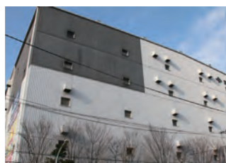
Ariake No. 3 ABC Center (Ariake, Koto-ku, Tokyo)
